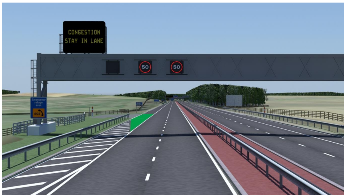
Figure 1 – Example of gantry mounted variable speed limit signing
