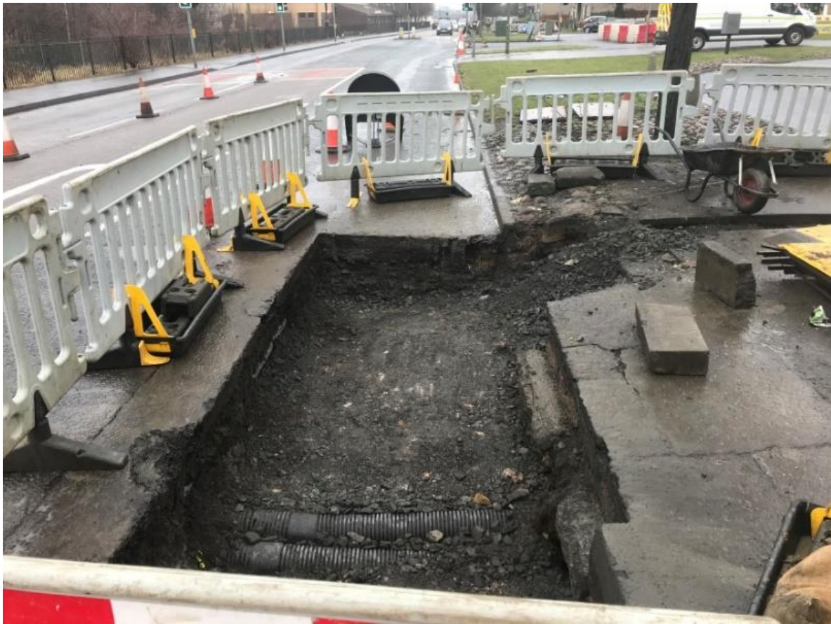
Figure 2 - Traditional trench methods showing a large exposed area
