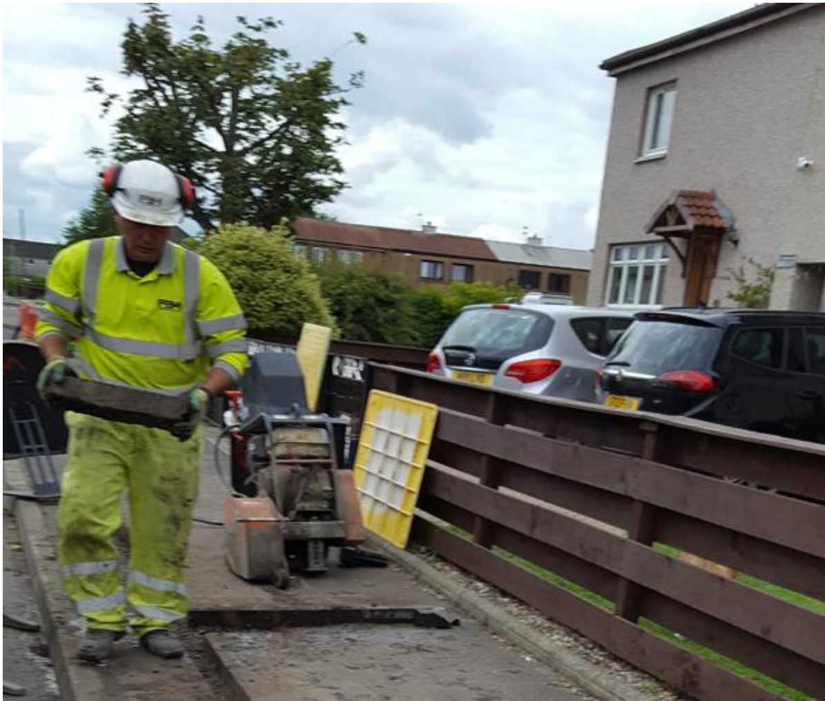
Figure 1 - Operative standing on a traditional pavement, beside a 100 mm narrow trench
